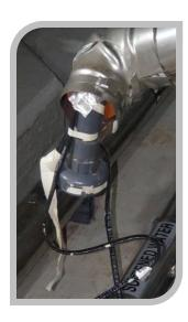
As part of advanced storm preparation, SAWS utilizes heat tracing which is to insulate critical small diameter piping subject to freeze impacts with electric heat tapes.
