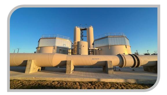
The SAWS Agua Vista Station at sunset, looking at the lime silos with saturator tanks.
