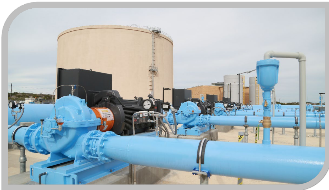
One of the storage tanks and high service pumps at the Agua Vista Station which pumps Vista Ridge water into SAWS distribution lines
