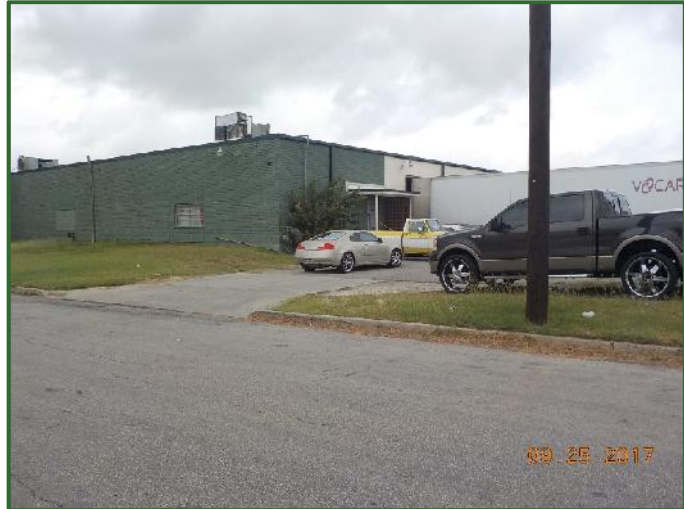
PHOTOGRAPH #4 – REC #1 Turbine Support, located at 4415 Dividend Drive.
